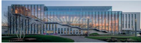
Believe in Better Building, London, UK
