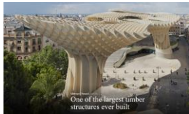
Metropol Parasol, Seville, Spain
